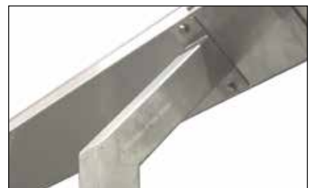
Central Cable Trunking
