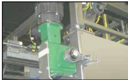
Main Carriage Drive
